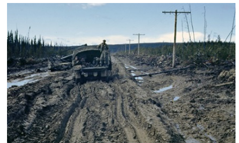
The mud was deep in the spring of 1943. This muddy section of the Alaska Highway shows the importance of proper drainage. Credit: Yukon Archives, Phillip Neal Fonds, 93/9 #46.
