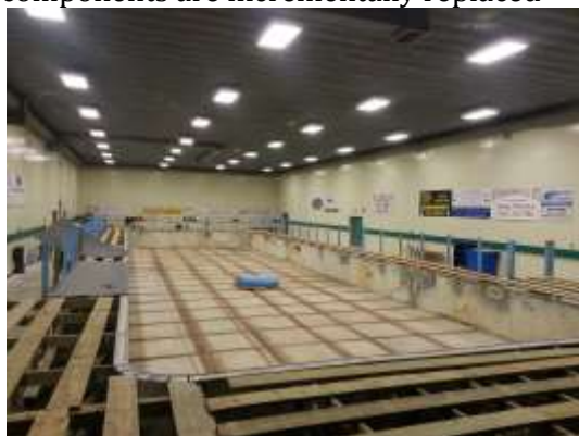
Pool being erected
