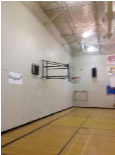
Interior second gymnasium
